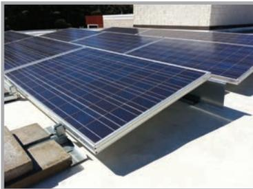
**Ballasted Roof Mounts
